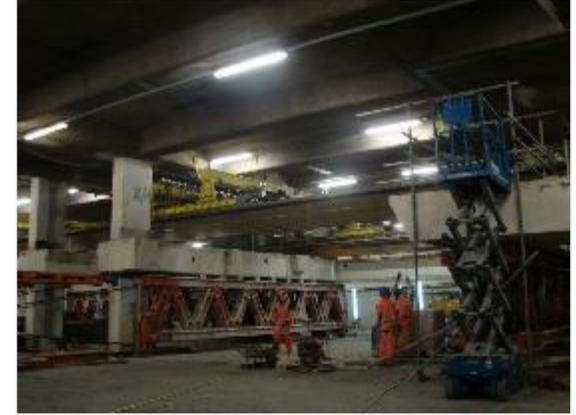
Mega Girder 3.6m – 14m Clear Span Working Range
